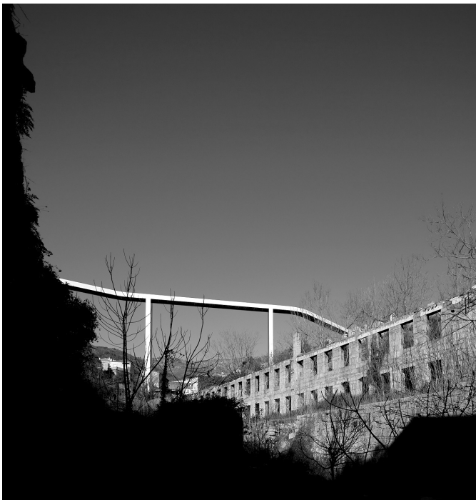
084 - The Covilhã Bridge.
