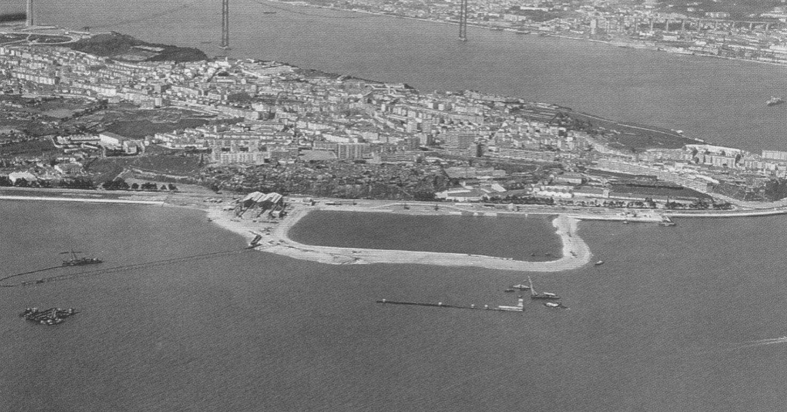
FIG 7, Lisnave in construction
