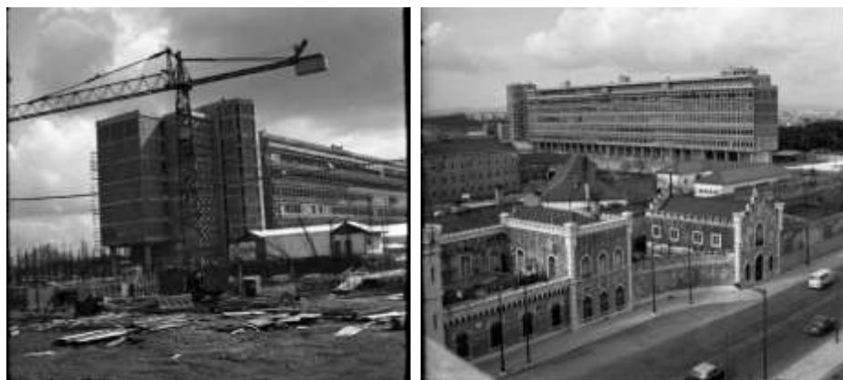
Figure 7 – Construction of Palácio da Justiça in Lisbon, 1969 (Source: Lisbon Municipal Archives | (left) Palácio da Justiça under construction, Artur Inácio Bastos, AIB002260; (right) Palácio da Justiça and Penitentiary, Artur Inácio Bastos, A66398).
