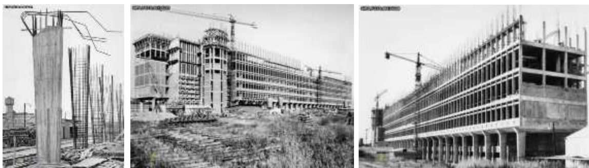
Figure 6 – Construction of Palácio da Justiça in Lisbon, 1968 (Source: SIPA/Forte de Sacavém).
