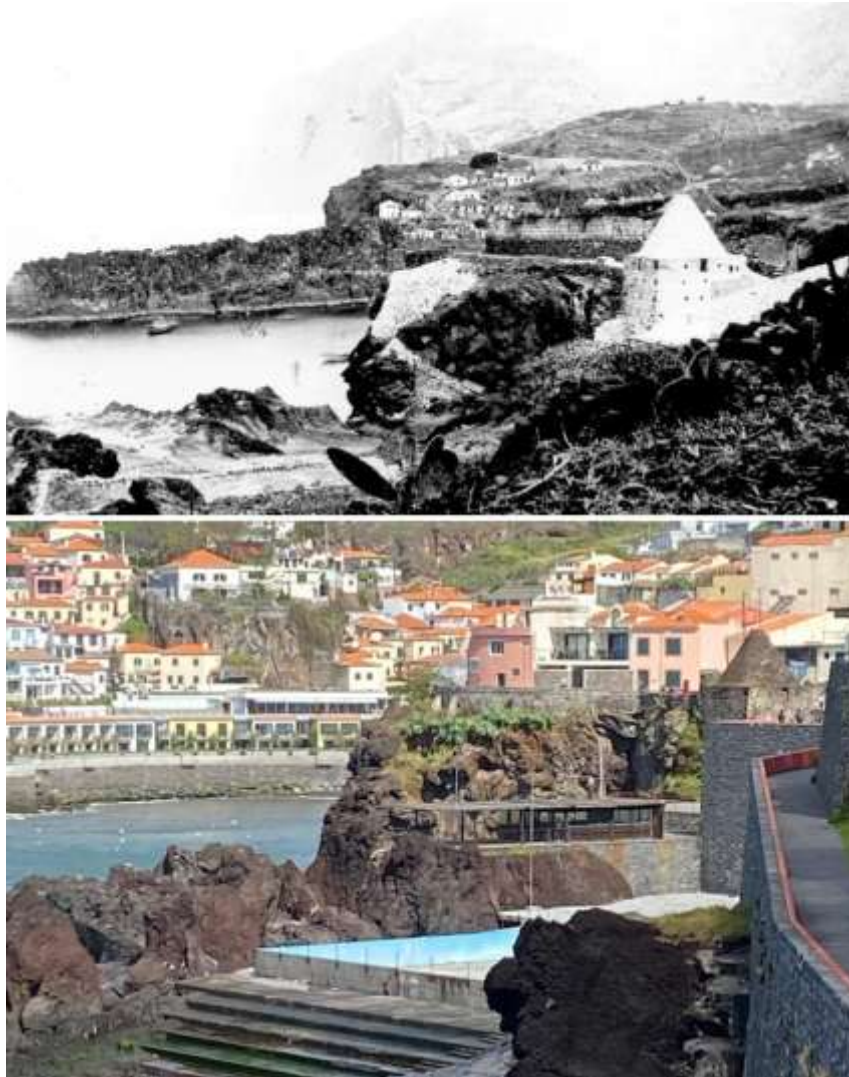
Figure 35 (top) – Photo of the salt pans and the bottom of the lime kiln are located in Trincadeira, above the old salt pans, in the parish of Câmara de Lobos, and were built around 1874 by Roque Teixeira de Agrela. (Source: Madeira Library Collection. Available at: https://arquivo-abm.madeira.gov.pt/descriptions/73569 [Consult. June 2026]). Figure 36 (bottom) – Pool Bar. Sunbathers. Photo by Pedro Kok. (Source: Available at: https://www.pedrokok.com/salinas-complex-at-camara-de-lobos-madeira-portugal/ [Consult. June 2026]).
