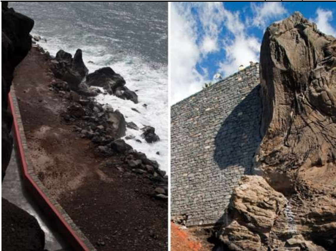
Figures 13 and 14- Two Photos by Leonardo Finotti. You can see the promenade and the wall. The structural part of the concrete is painted in oxide red, the sidewalk in raw concrete, with basalt coating and, in the background, the natural stones and the sea (Source: Available at: https://landezine.com/salinas-swimming-pools-by-global-arquitectura-paisagista [Consult. June 2026]).
