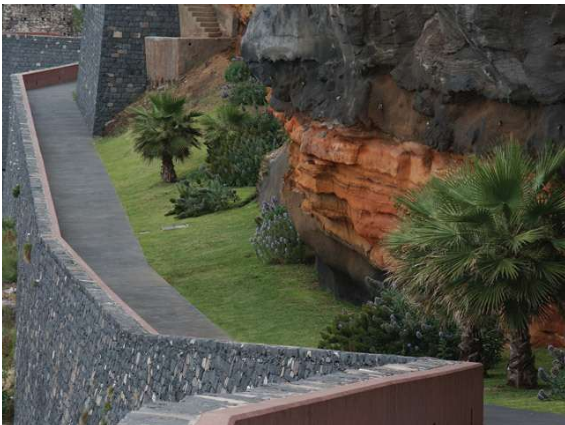
Figure 10 - Image of the Wall part of the Promenade. Photo by Martin Sauter. You can see the rocky wall and its mineral layers (Source: Available at: https://landezine.com/salinas-swimming-pools-by-global-arquitectura-paisagista [Consult. June 2026]).
