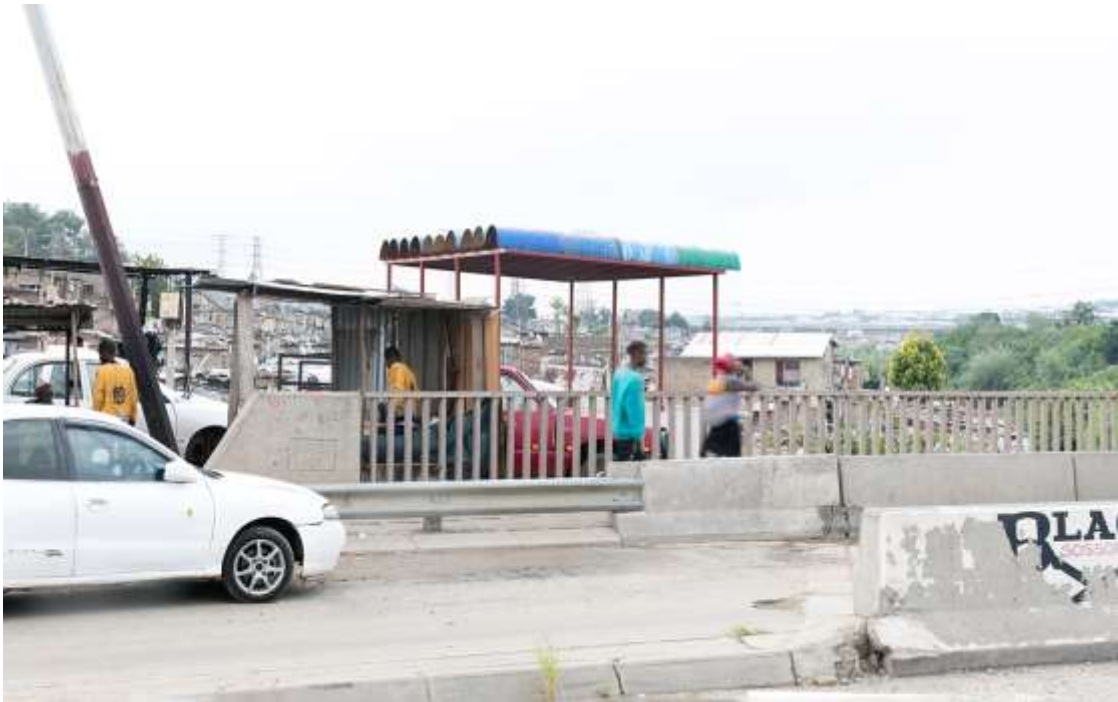
Figure 13 – The impactful roof structure of the Southern shed, made from repurposed 44-gallon drums, draws attention while creating pleasant shade. The space is used by the K Stjwetla Patrollers and the community in general (Credit: Leon Krige).
