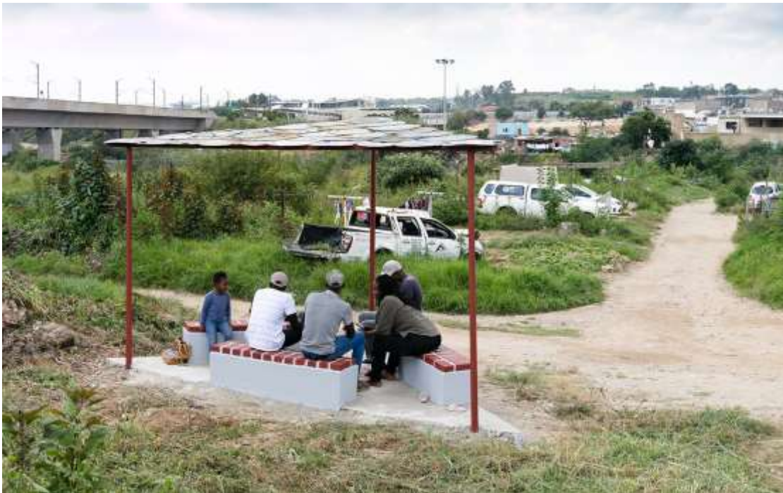
Figure 11 – The roof of the northern shelter incorporates the lids from the same drums used in the southern structure, demonstrating the possibility of reusing 100% of the material with zero waste. The actual shelter is triangular in form, with an unwall platform with three benches creating a space for gathering, encouraging dialogue and social interaction (Credit: Leon Krige).
