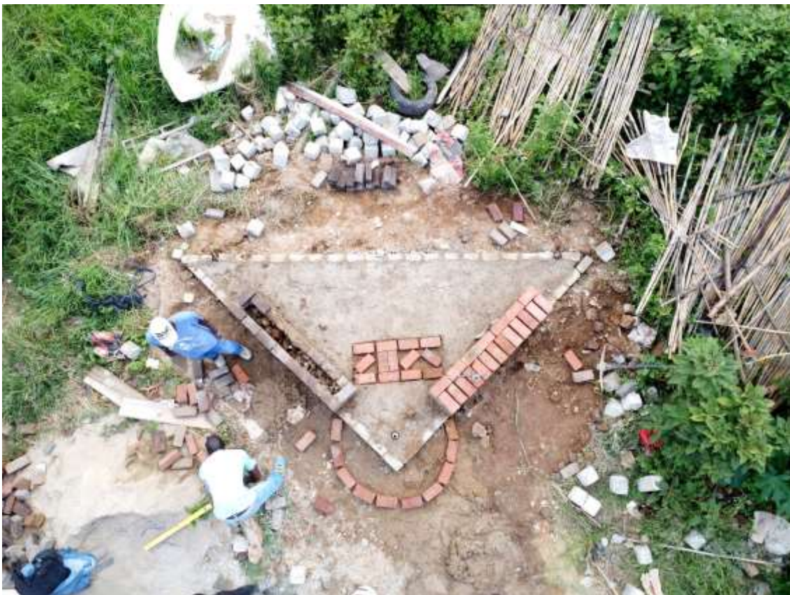
Figure 10 - In February and March 2025, a small team of four local artisans and builders worked to construct the Northern shelter, with a triangular shape (Credit: Michael Tinapi).
