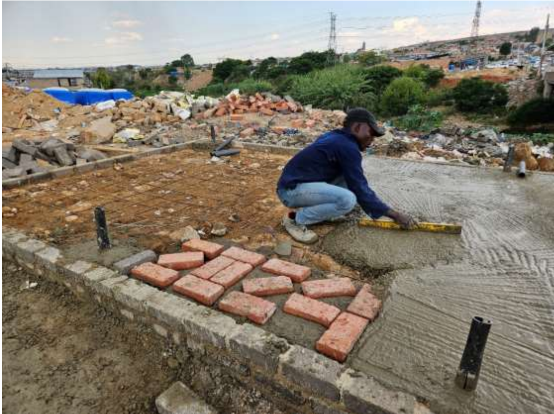
Figure 12 - In November and December 2024, a team of ten local artisans and builders worked to construct the southern shelter using recycled materials where possible (Credit: Paulo Moreira).
