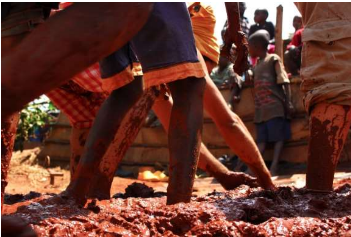
Figure 7 – WNA, fase 2 – earth preparation
