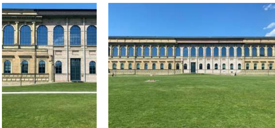
Figures 12 and 13 – Alte Pinakothek, Leo von Klenze (1826-37) and Hans Döllgast (1946-57), south façade, Munich (Source: author's photograph, 2022).
