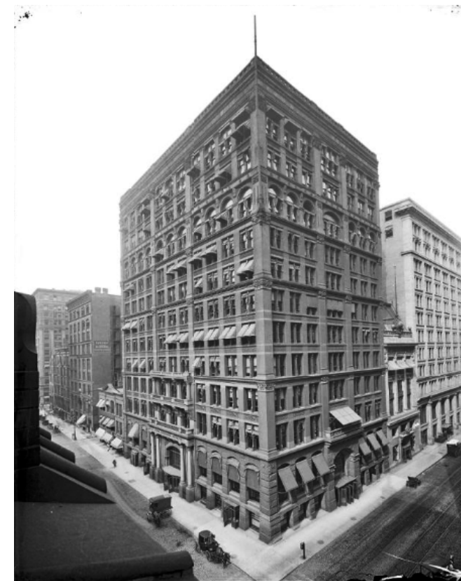
Image 120. W.L. Jenney's Home Insurance Building, LaSalle and Adams Streets [Photograph]. (1995).
