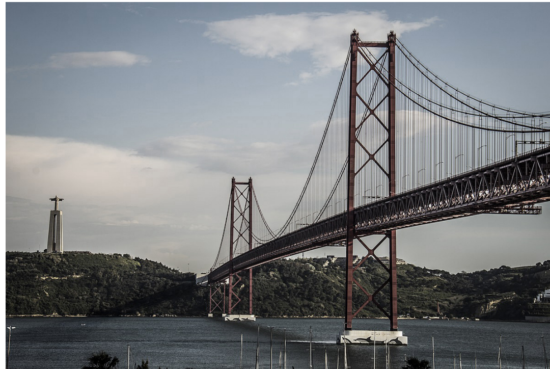
Image 78. Alcântara, 25 de Abril Bridge [Photograph].(2018).
