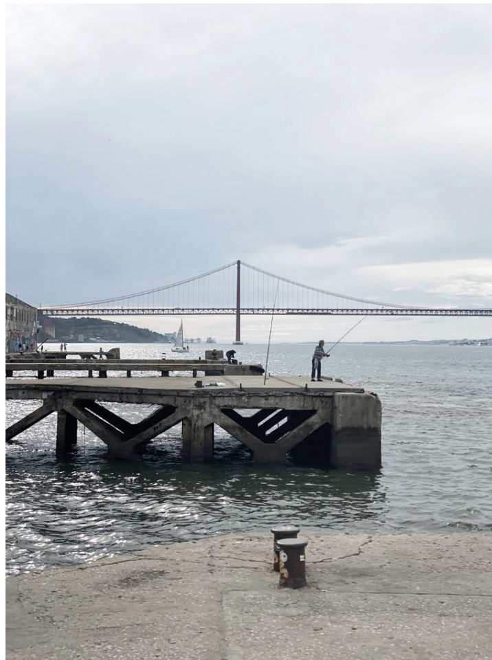
Image 32. Concrete piers in Ginjal [Photograph] (2021).
