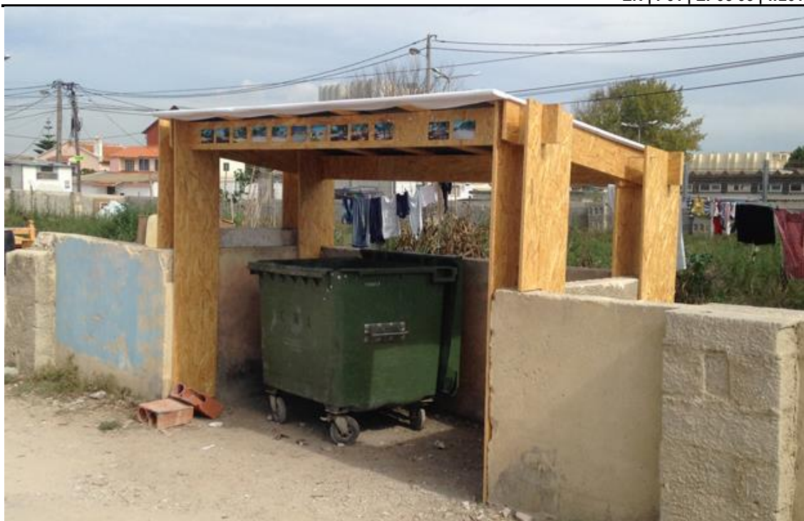
Figure 12 – (4a) Waste management, cover for a container.
