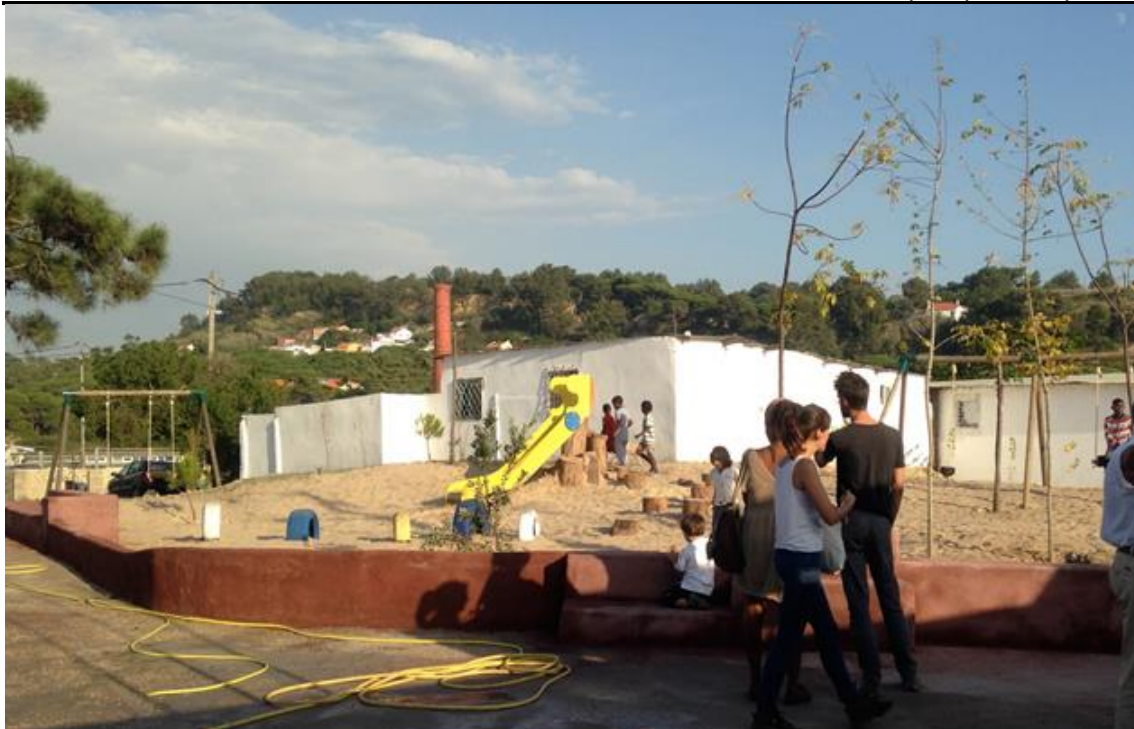
Figure 23 – (1) Largo do Café Convívio, playground. Last day of construction of InSituAction.
