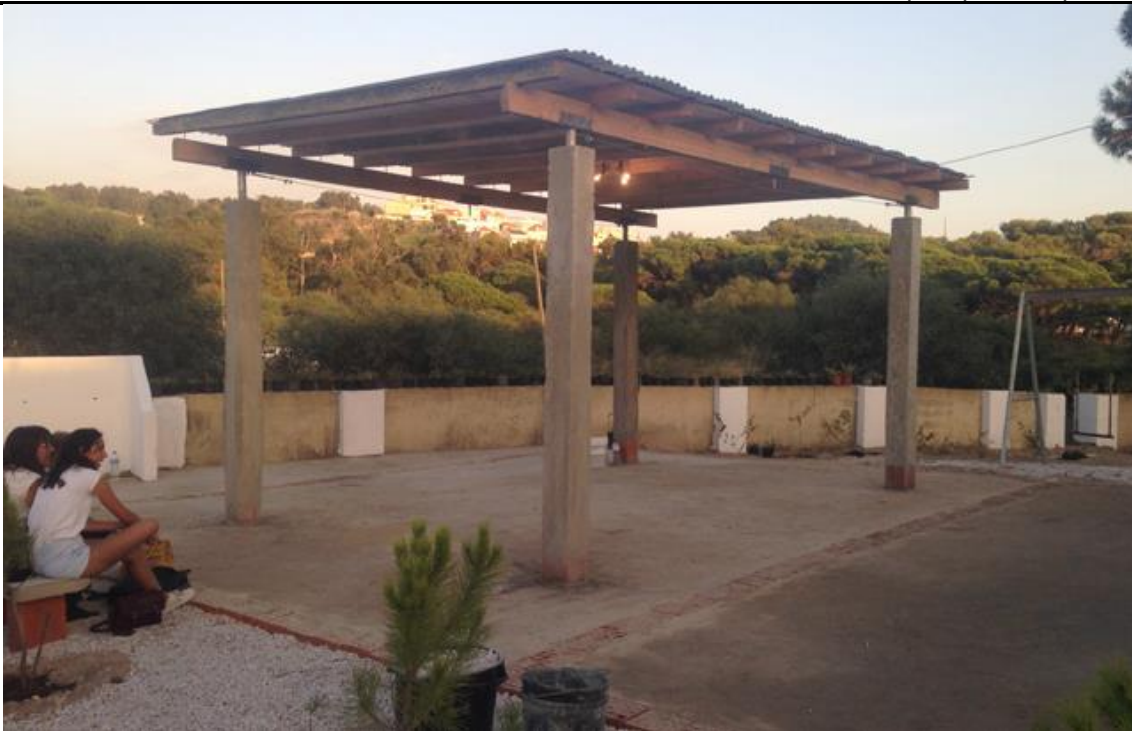
Figure 26 – (2) Side space next to the Residents' Association. Last day of construction of the InSituAction.
