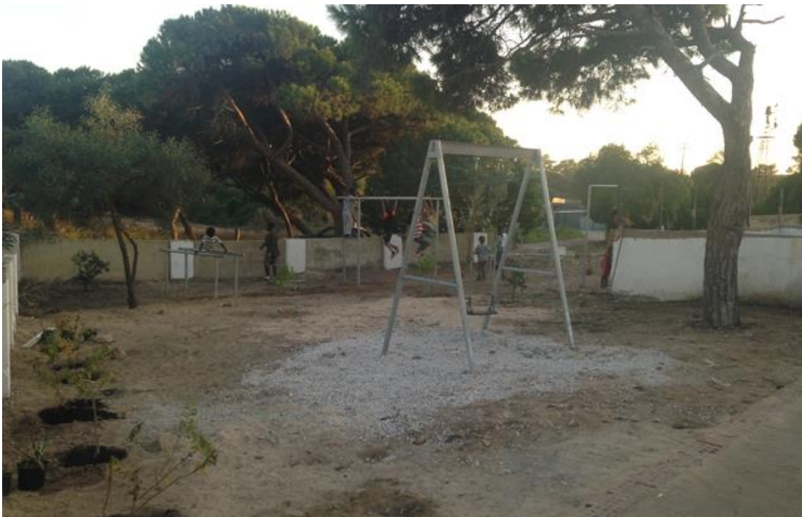
Figure 27 – (2) Outdoor exercise area. Last day of construction of the InSituAction.
