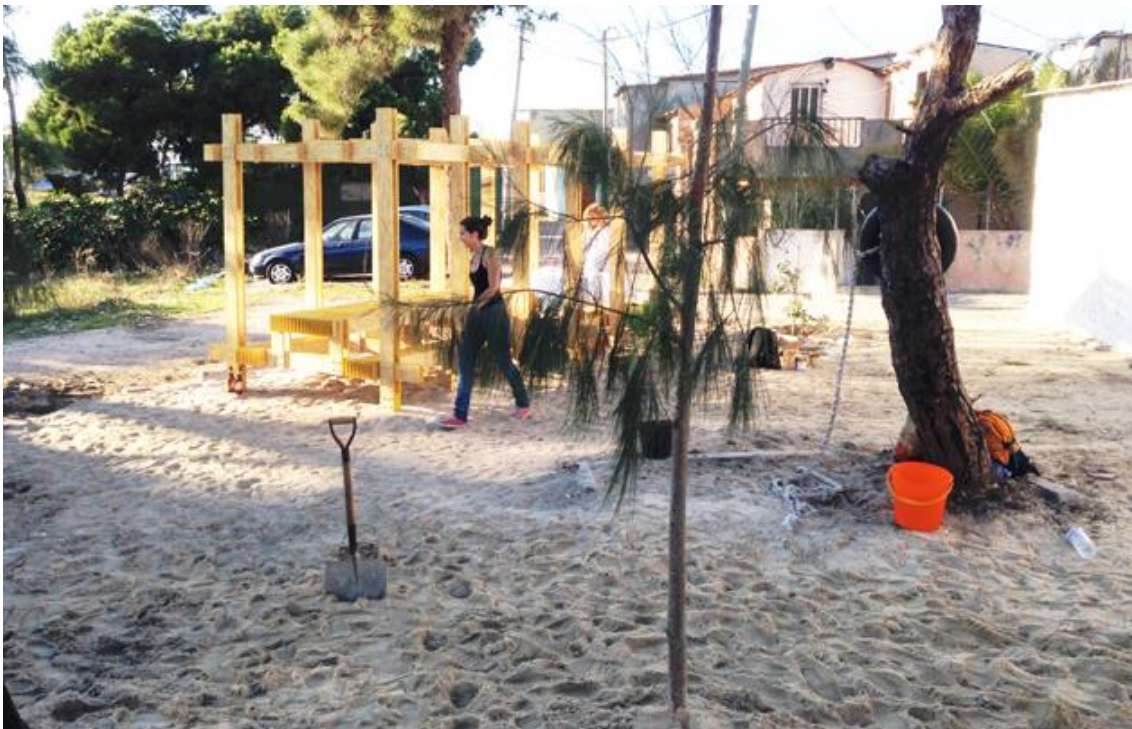
Figure 8 – (2) Gathering space with the table and potential garden on the final day of construction during the InSitu Lab.
