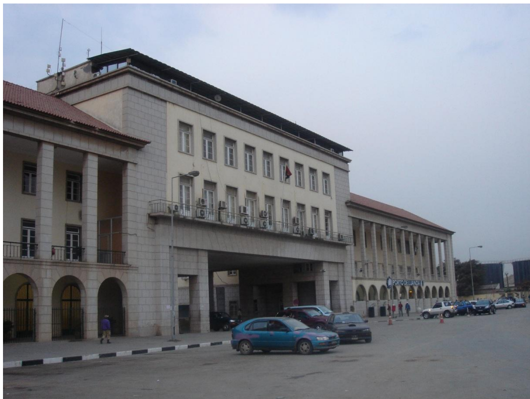
Fig. 16: Facilities of the port of Luanda, Eurico Pinto Lopes/CUO 1948. Photograph: Ana Vaz Milheiro, 2009
