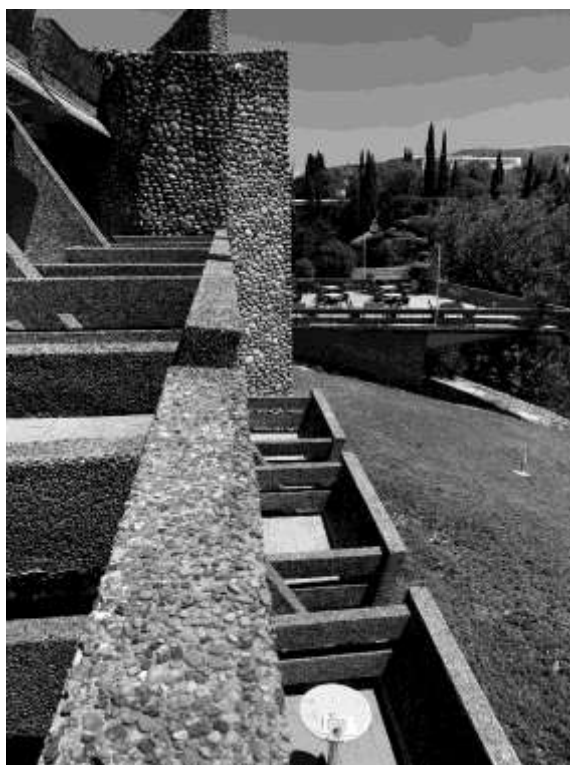
Figure 17 - Surface texture of the concrete façade at Hotel Podgorica. (Source: Photograph by the author, 2025).
